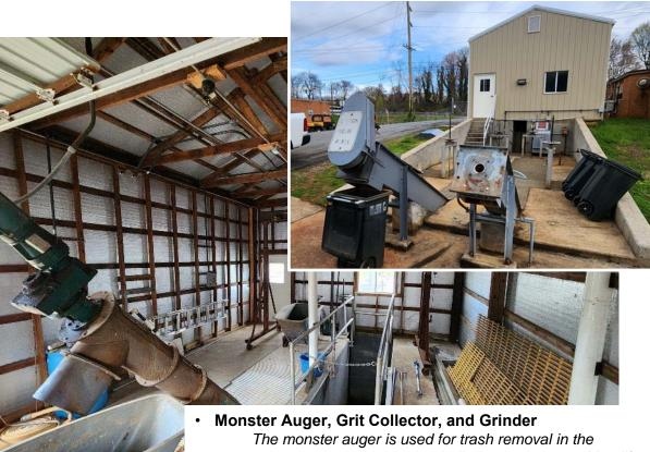
The monster auger is used for trash removal in the treatment process. It was rebuilt two years ago, with a life expectancy of two years before complete replacement would be necessary.
