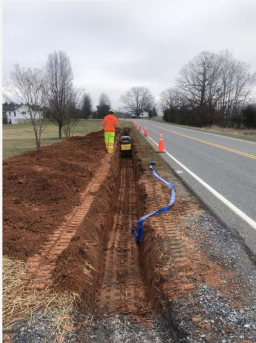
Work on the waterline continues.
