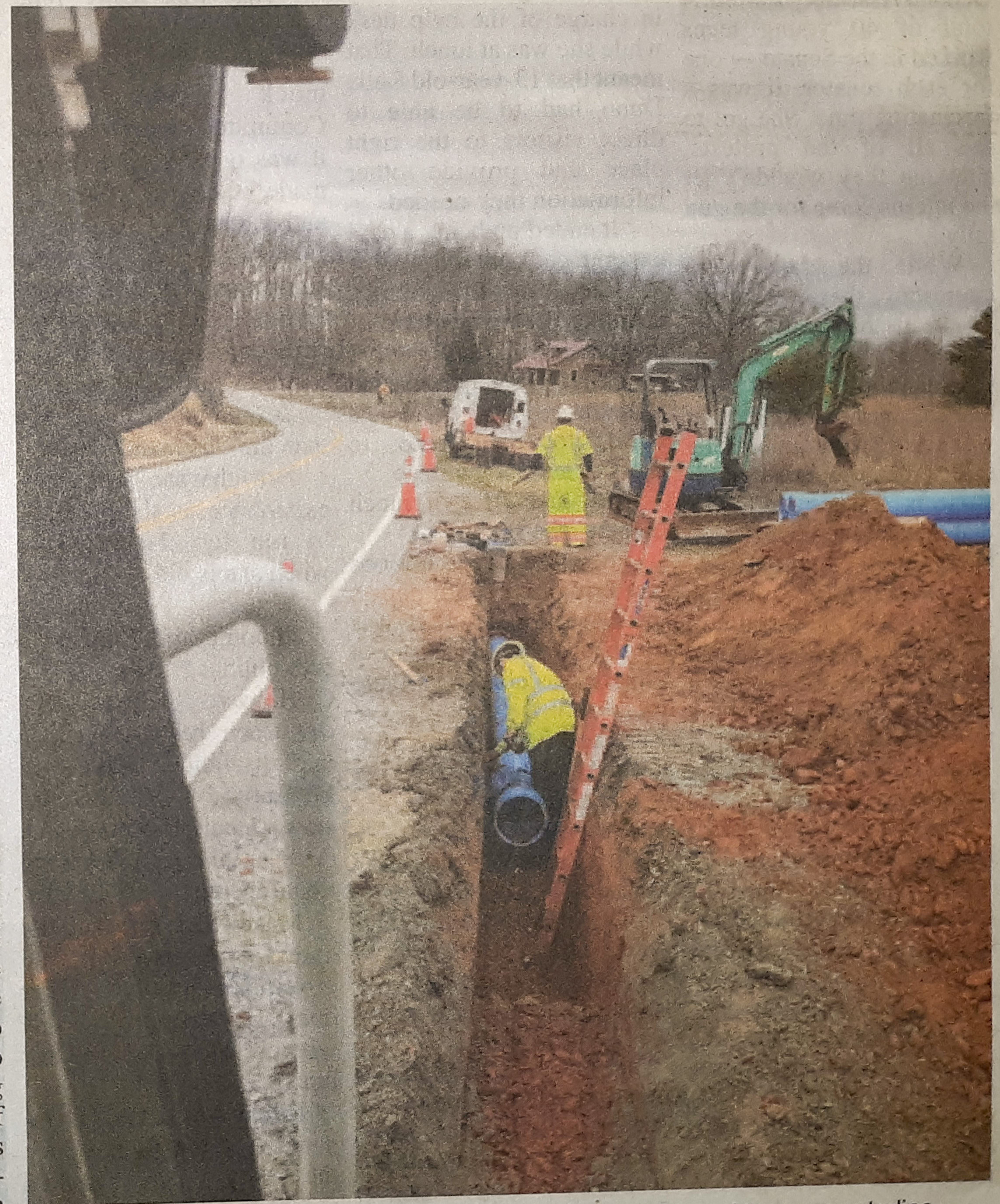
The Authority CIP Maintenance Team installing a section of the new waterline.
