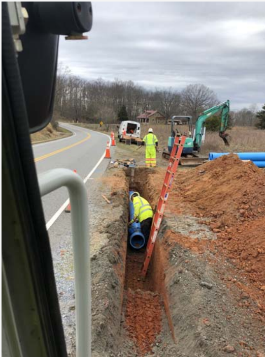
The Authority CIP Maintenance Team installing a section of the new waterline.
